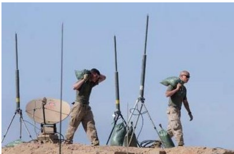
U.S. marines work on trenches during a visit by government officials in Marjah city, Helmand province, March 1, 2010. REUTERS/Massoud Hossaini/Pool
